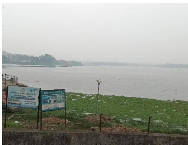
FIG -3 KANKE DAM
